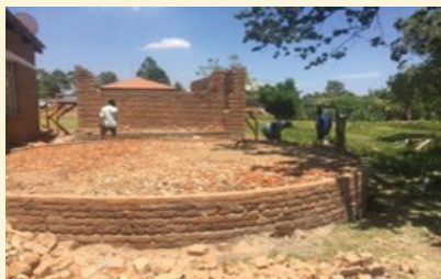
Constructing our building in Malawi
